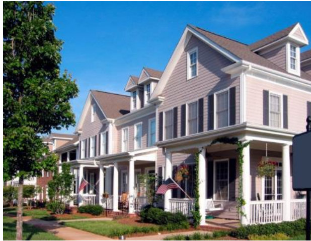
Figure 9.03-A: This image illustrates how multiple design features are incorporated into the design to de-emphasize the fact that this is a single structure.
