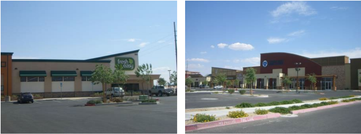
Figure 9.04-E: An example of dynamic roof lines
