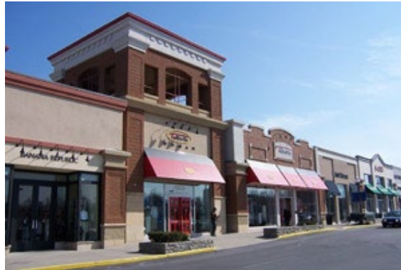
Figure 9.04-B: The above image illustrates a building that contains pilasters, cornices, and a series of façade setbacks (recesses) to visually break up the appearance of the large facade.
