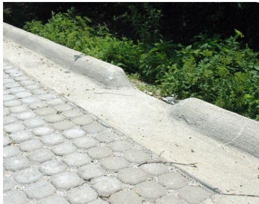
Figure 11.03-A: Cuts in the continuous curb allow for stormwater to be directed into landscaped areas.
