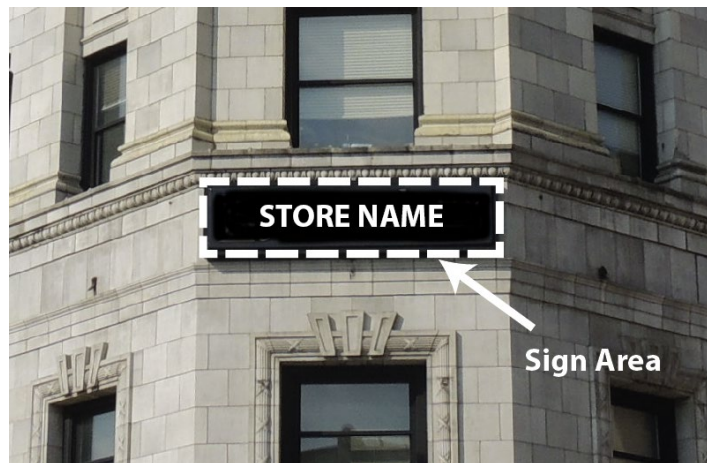
Figure 12.07-C: Illustration of computing the sign area for wall signs with a background panel or cabinet.
